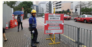
Notice with on-day blasting schedule
