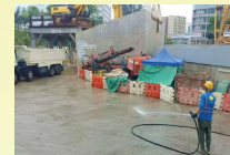
Spraying water to reduce dust
