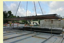
Covering the noise enclosure
