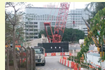
Installing noise barriers
