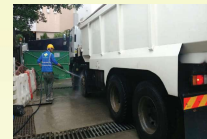
Washing the wheels of dump trucks
