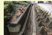
Cleaning up stagnant water
